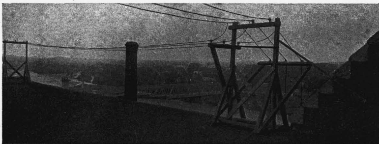
FIG. 18. SUBSTANTIAL WOODEN ROOF STRUCTURES.
