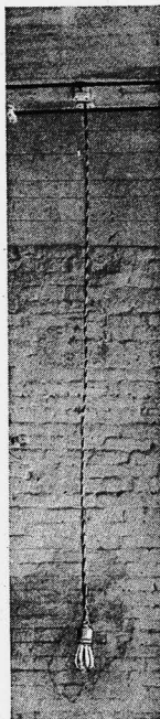
FIG. 42. LONG WATERPROOF PENDANT, WIRES TWISTED TOGETHER.
