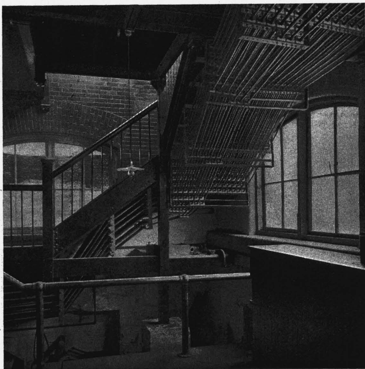
FIG. 8. LARGE GROUP OF WIRES, WELL SUPPORTED.
