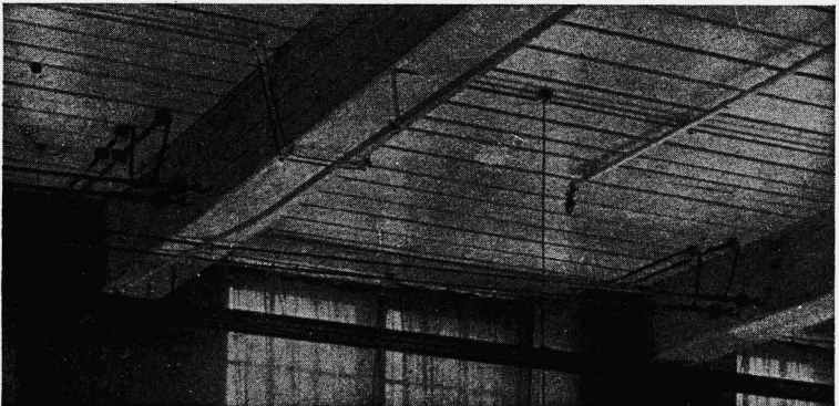
FIG. 33. OVERHEAD WIRING, SHOWING USE OF STRAIN INSULATORS.
