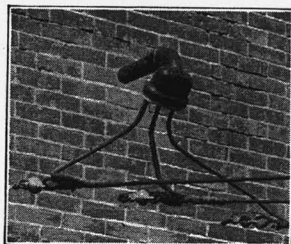
FIG. 21. WIRES ENTERING BUILDING THROUGH CONDUIT AND SERVICE HEAD.
