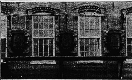
FIG. 29. TRANSFORMERS ON OUTSIDE WALL.
