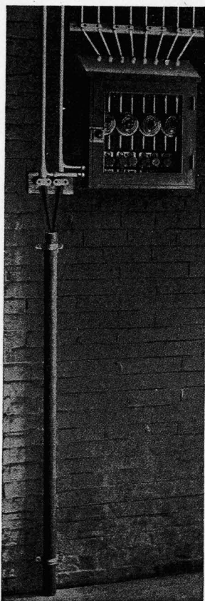
FIG. 45. CABINET WITH SNAP SWITCHES AND PLUG FUSES.
