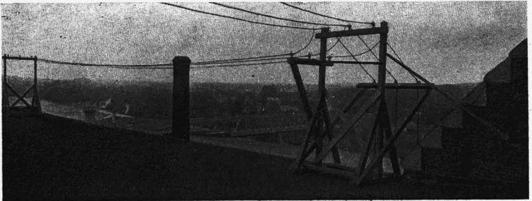
FIG. 19. SUBSTANTIAL WOODEN ROOF STRUCTURES.
