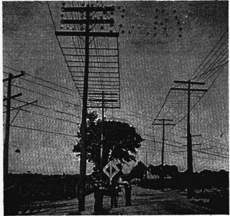
FIG. 26. CROSSING PROTECTED BY SCREEN.
