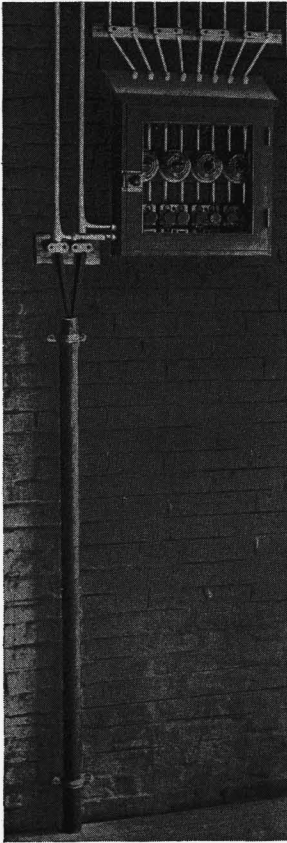
FIG. 44. UNLINED CABINET WITH SNAP SWITCHES AND PLUG FUSES.
