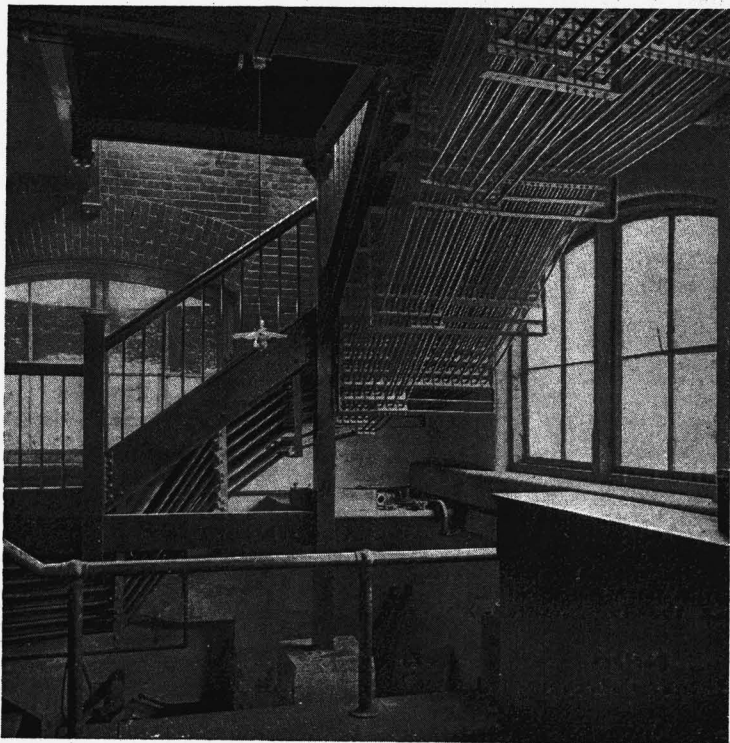
FIG. 8. LARGE GROUP OF WIRES, WELL SUPPORTED.
