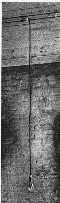
FIG. 42. PENDANT WITH REINFORCED FLEXIBLE CORD.
